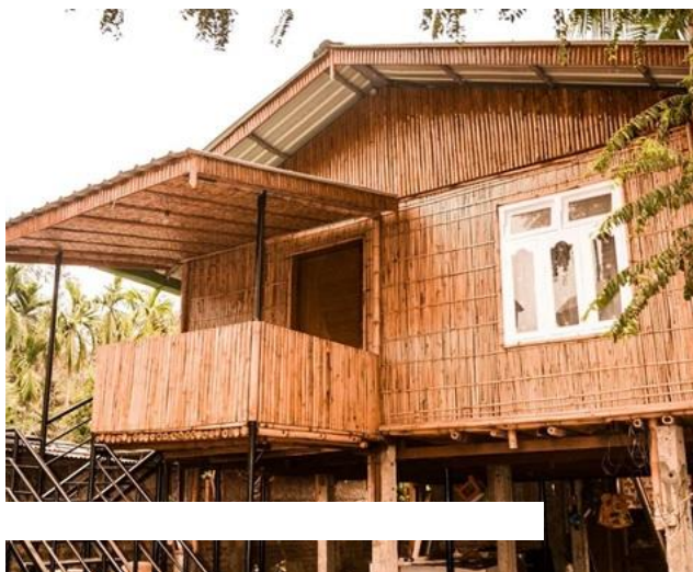
Figure 14 Residence in the City of Guwahati built on RCC stilts and Bamboo superstructure. Source: Author, Residence Designed for Mr. Dilip Narzary at Guwahati Assam by Ar. Kankana in the year 2015
