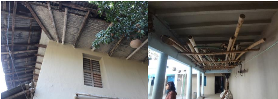
Figure 2.3, Structural Details of a Mud house in Kaligram
