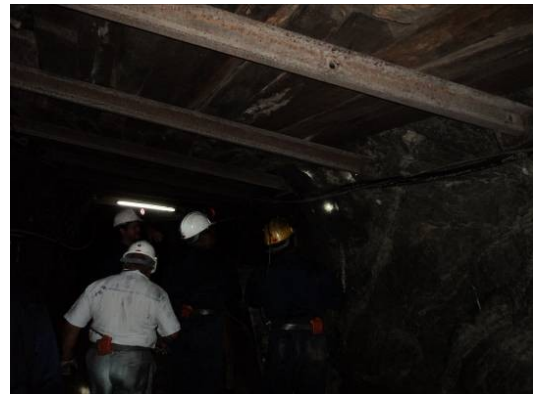
Figure 4: Roof fixing in Bogala. This was taken during a field visit to Bogala at main cross cut in 503m level.
