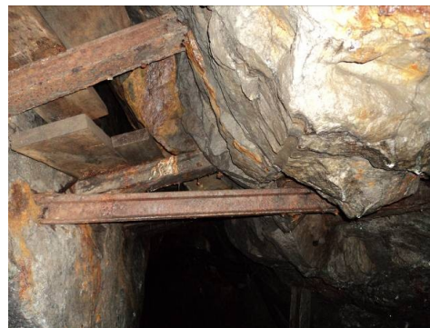
Figure 8: Heavy support system in Bogala. Heavily supported rock piece at Bogala in 260m level.
