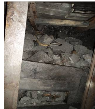
Figure 5: Side wall fixing in Bogala. This was taken at Na veins 2 nd working bench in 260m level.
