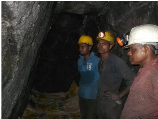
Figure 6: Open stope mining method at Ragedara. Unsupported working stope roof due to rock strength.
