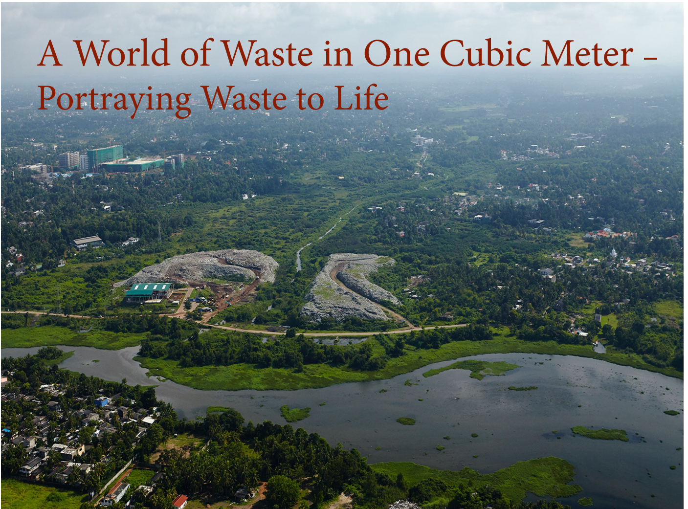
Figure 1: Aerial View of Karadiyana solid waste site – University of Moratuwa is in the background
